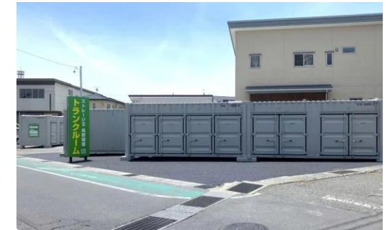
Nagano Inaba Trunk Room
