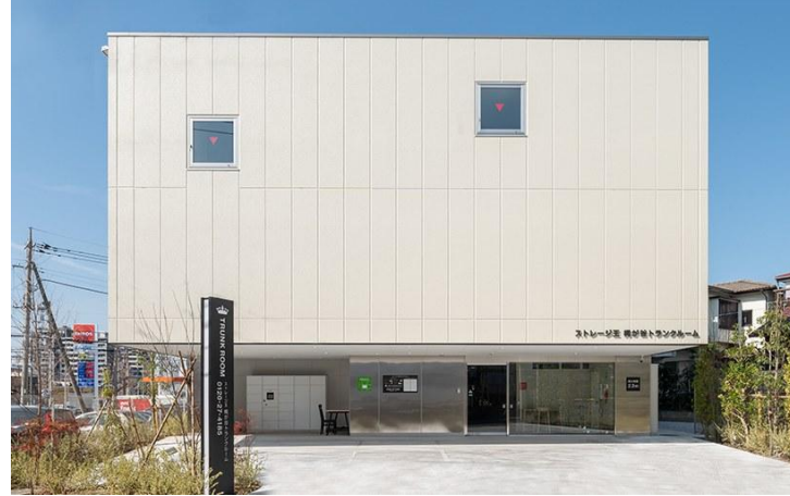
Kajigaya Trunk Room
