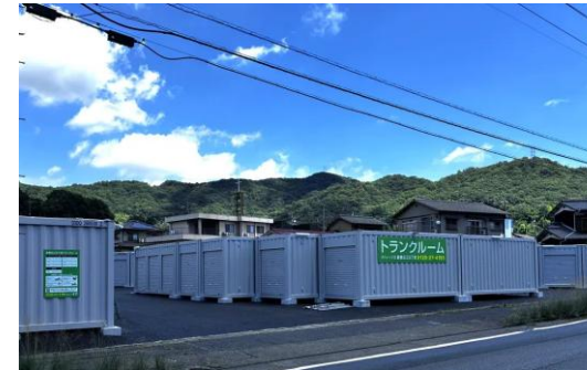
Kurashiki Hiroe 5-Chome Trunk Room
