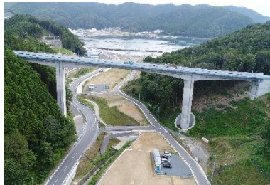
New bridge construction
